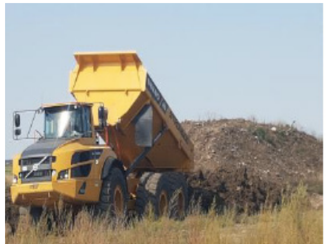
Haul truck unloading unloading soil – SF 28 – Sept 7, 2018
