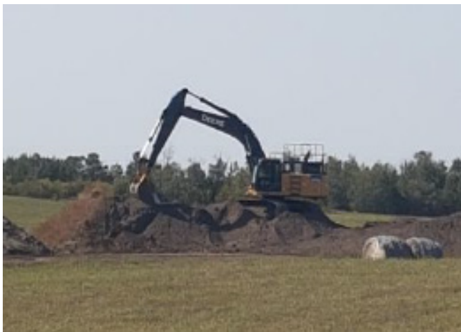
Excavator putting topsoil on ROW – km 32+500 - Sept 7, 2018
