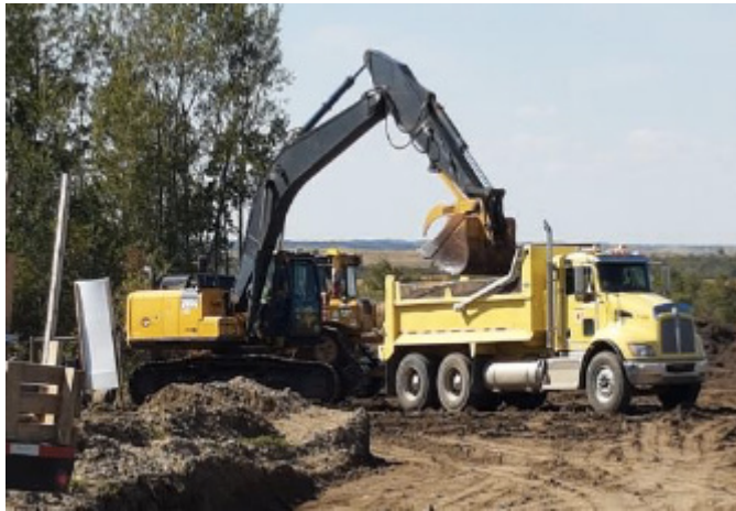
Excavator loading rocks onto haul truck – SF 21 - Sept 5, 2018
