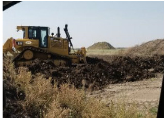
Dozer pushing soils on ROW – SF 28 – Sept 7, 2018
