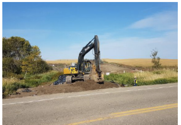
Removing ramp access – SF 26 – Sept 6, 2018
