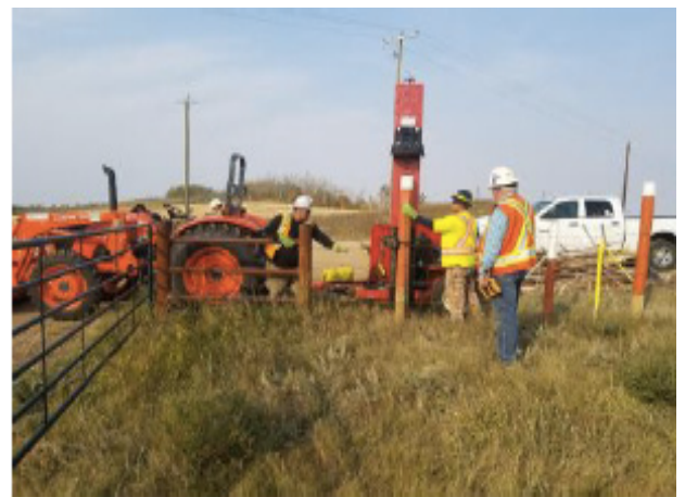
Post pounding, crews fencing – SF 7 –Sept 8, 201
