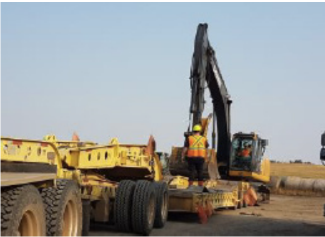
Excavator being loaded unto lowboy – SF 27 – Sept 8, 2018
