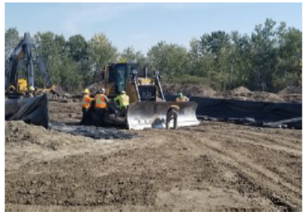
Crews rough cleaning dozer – SF 21 – Sept 5, 2018
