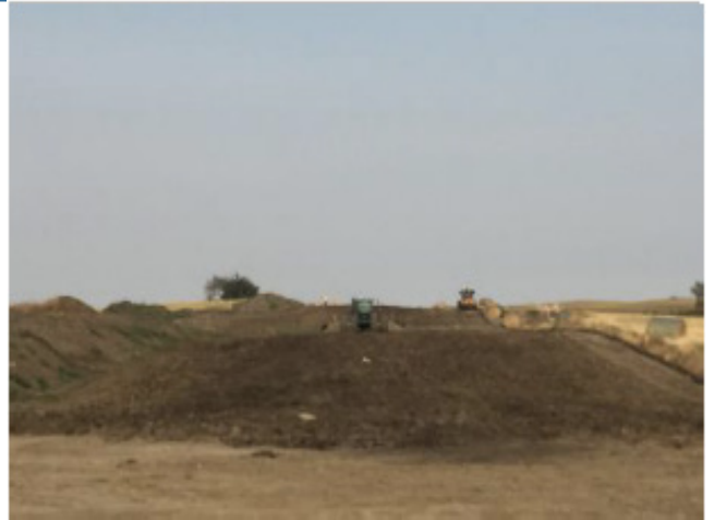
Harrowing and dozer subsoil – km 35+500 - Sept 8, 2018
