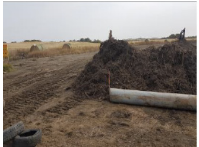
Culvert removed from access – SF 23 – Sept 8, 2018
