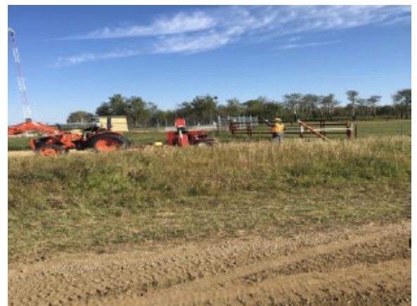
Utility Crew fencing - SF 9 - Sept 5, 2018
