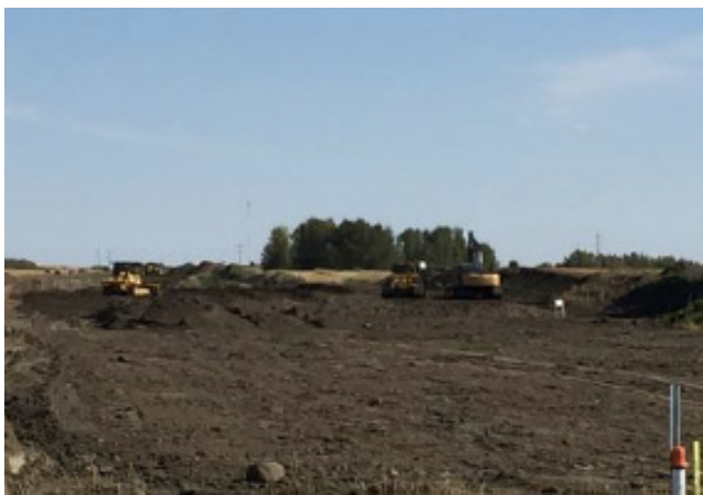
Dozer and excavator shaping subsoil - SF 23 - Sept 5, 2018
