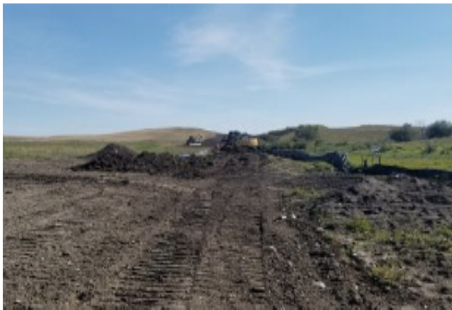
Excavator wetland ramp removal – km 30+200 - Sept 5, 2018
