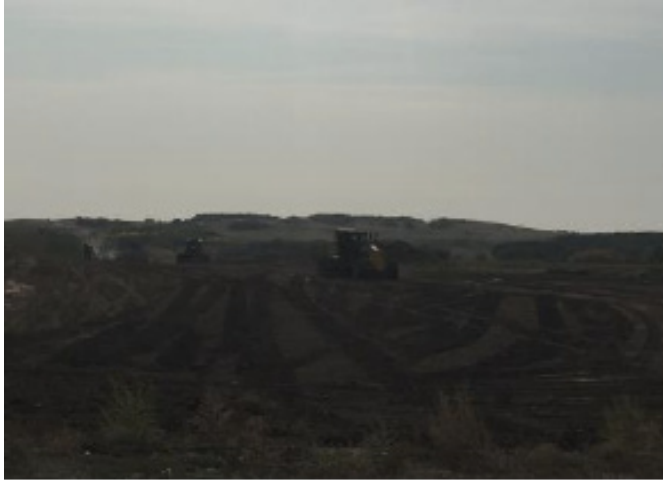
Dozer and grader working on subsoil- SF 28 – Sept 8, 2018
